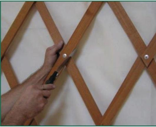
Center the stovepipe outlet on a rivet in the lattice wall approximately 56" above the floor. This may be a little higher or lower based on the height of your stove the length of your stove pipe, but should be centered on a lattice wall rivet.
