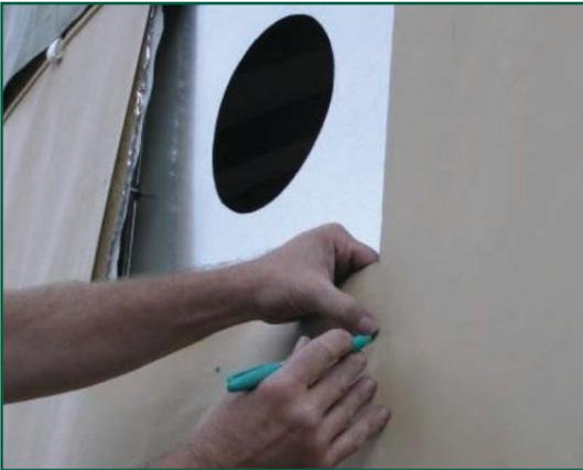
Mark the eight bolt holes and poke holes through the fabric using one of the sheet metal plates as a template. Poke through the fabric with a nail or other sharp object.
