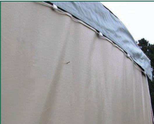
Poke a hole through the fabric wall at the center mark of the lattice opening you just cut out. Use a nail or other sharp object. This will allow you to determine the center of the stovepipe outlet from the outside of the yurt.
