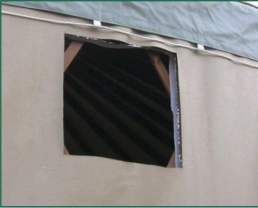
Cut and remove an 18"x18" square of fabric centering the square over your nail hole. Use scissors or a utility knife. If you have insulation, cut the fabric, insulation and insulation liner fabric separately.
