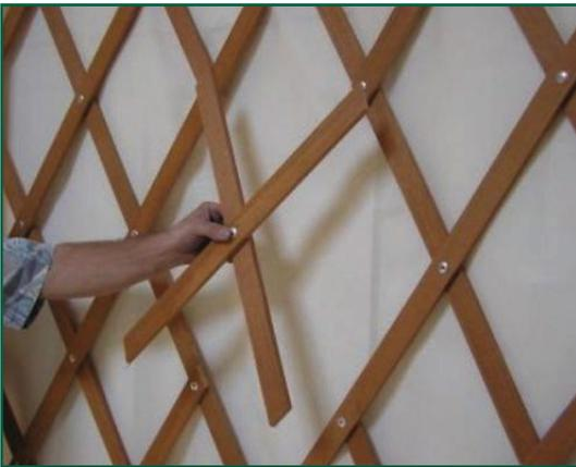
Cut and remove the lattice pieces around the center rivet using a small hand saw. Cut flush with the next crossing piece of lattice. You will be removing an "X" from the lattice wall
