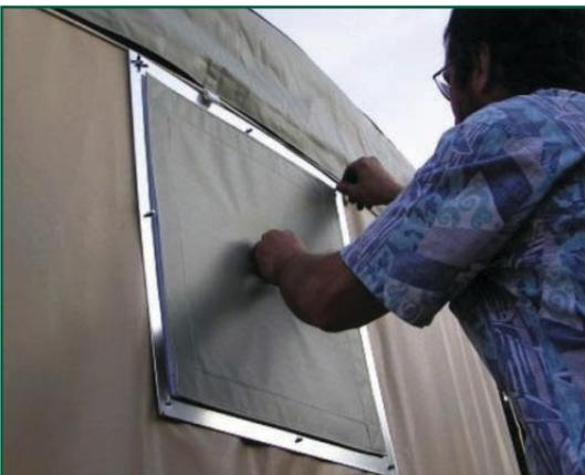
Push the bolts through the eight bolt holes in the fabric from the inside of the yurt.
