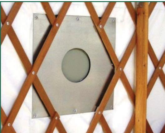
Place the other sheet metal plate over the bolts from outside the yurt and secure with the wing nuts provided. There will be an x marked in one corner of the inside sheet metal piece and the outside sheet metal piece of your stovepipe outlet. Make sure you match these two corners up when you place the outside piece on the bolts.
